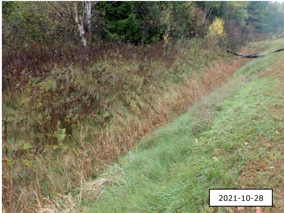
Channel identified as a roadside ditch with near uniform channel geometry. Riparian vegetation consisted of grasses and hardwoods.
