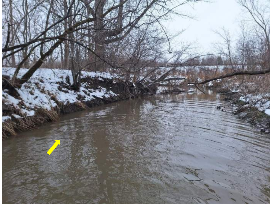
Channel transitions to a woody riparian edge. No riffle-pool formations observed. Slumping and scour observed.
