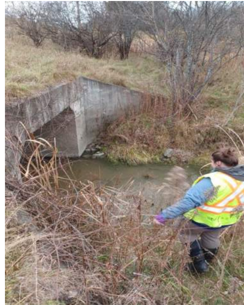
Existing conditions at Crossing 16 on the south side of Russell Road. Left photo is facing south, upstream; right photo is facing southeast. Some slumping was observed..
