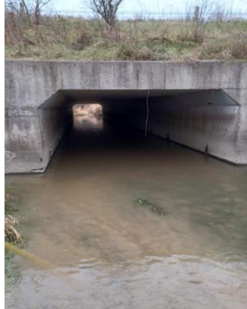
Existing conditions at Crossing 16 on the north side of Russell Road. Left photograph is facing north, downstream; right photograph is facing south, into the culvert. Some slumping was observed.
