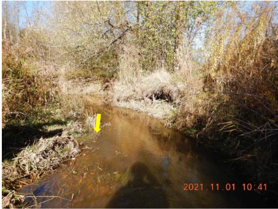
The featured conveyed flows through a woodlot, riparian vegetation consisted of mature trees. Slumping, undercutting and scour common.
