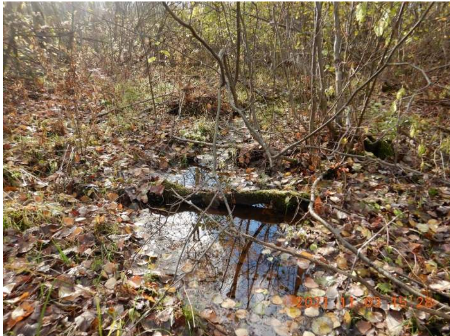
The feature was defined with multiple culverts throughout the reach. Riparian vegetation consisted of grasses and small hardwoods.
