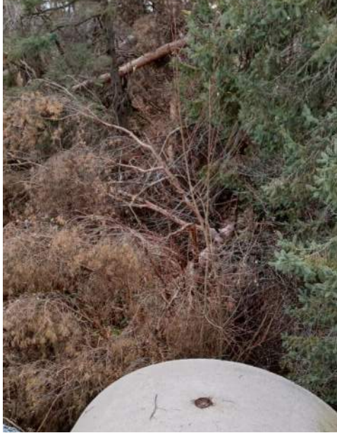
Existing conditions at Crossing 32 on the west side of Ramsayville Road. Left photo is facing west, a large number of down trees from recent storm are present in the channel; right photo is facing down at the mouth of the culvert. An erosion scar was observed on the left bank.
