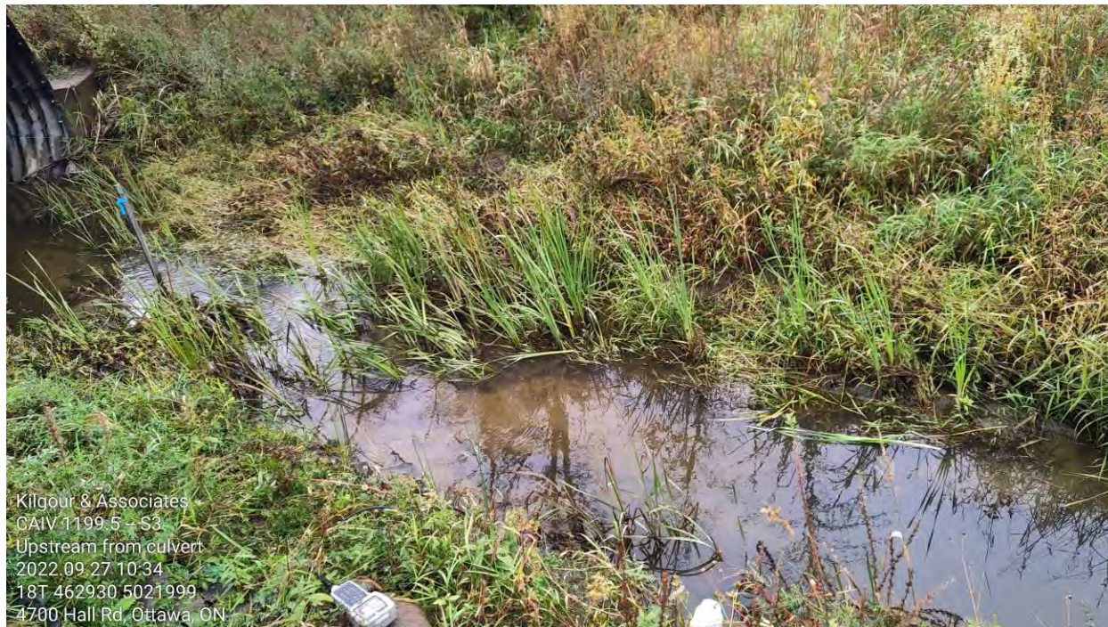
Figure 53 Photograph of the culvert inlet at S3 (photo taken on September 27, 2022)
