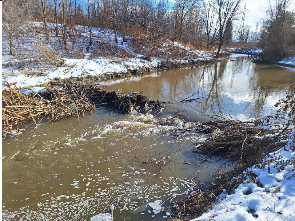
A large beaver dam was observed towards the downstream extent of the reach, causing backwatering. Extensive evidence of beaver activity was observed throughout the reach.
