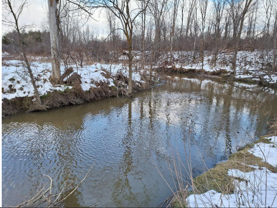
Undercutting was observed at two locations along the reach, concentrated along inside banks. Exposed tree roots were commonly observed.
