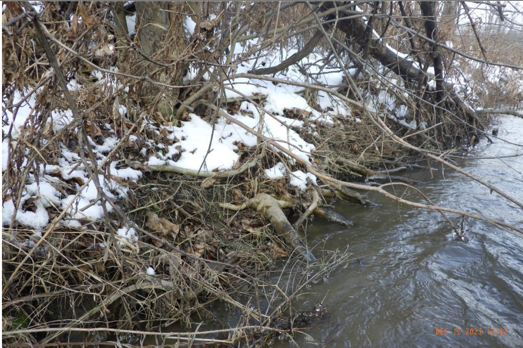
Exposed roots were observed throughout the reach as were fallen and leaning trees.
