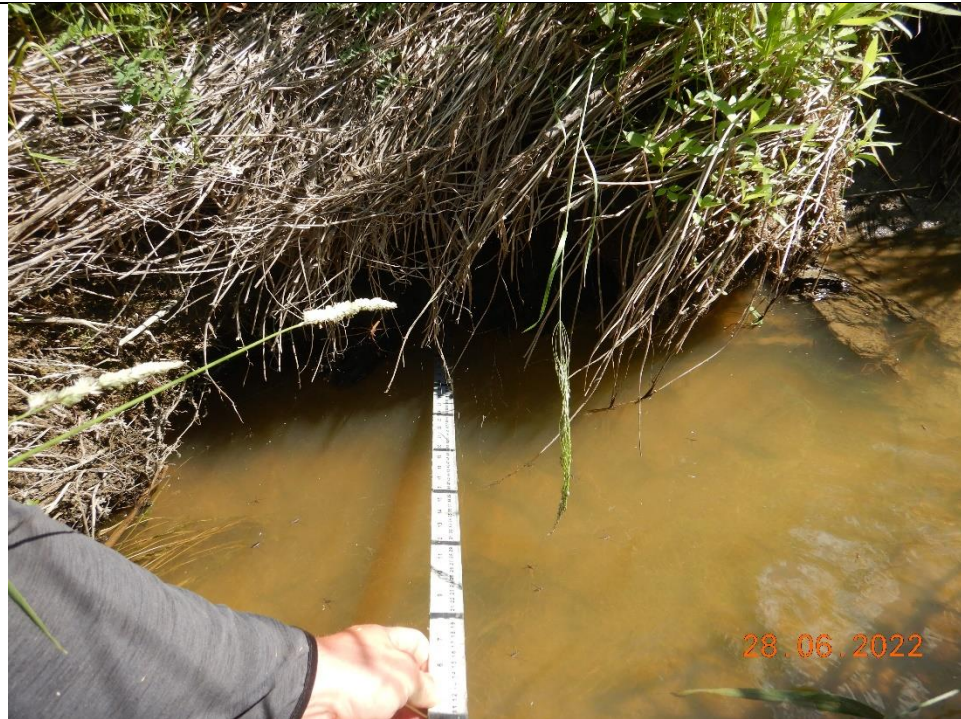
Channel bank slumping and undercutting were observed frequently.
