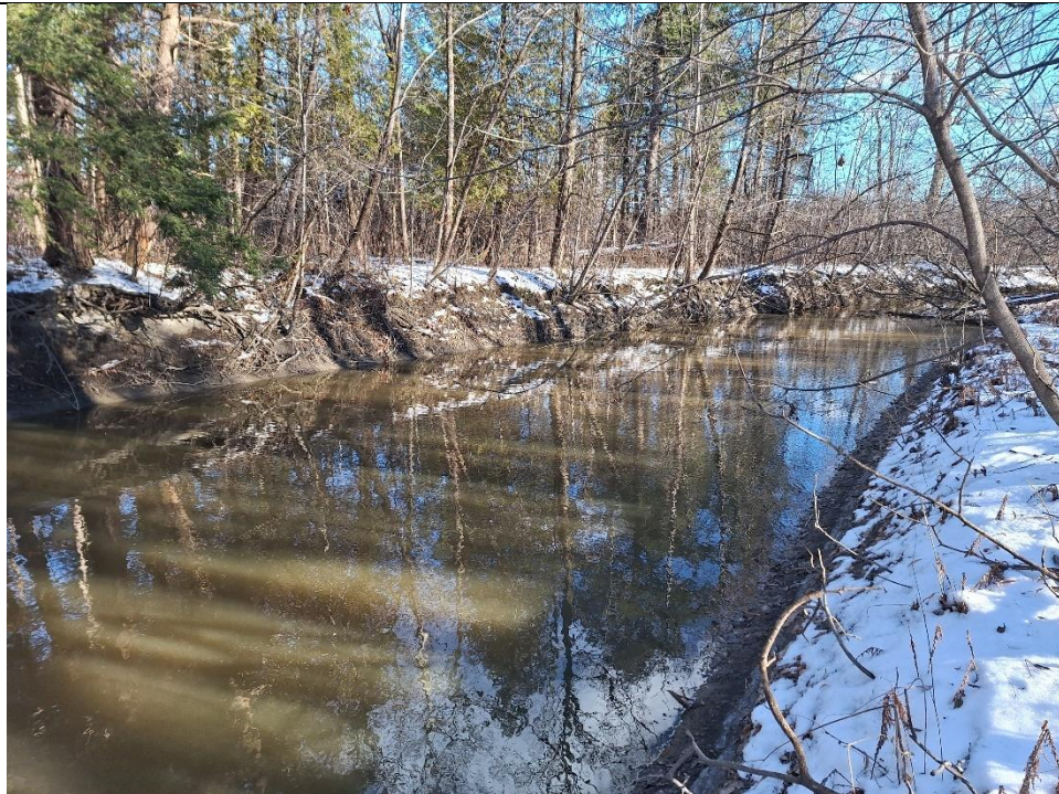
The downstream extent of the reach exhibited a straight planform and tall vertical banks.
